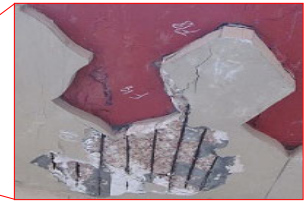
Severe corrosion due to low pH
